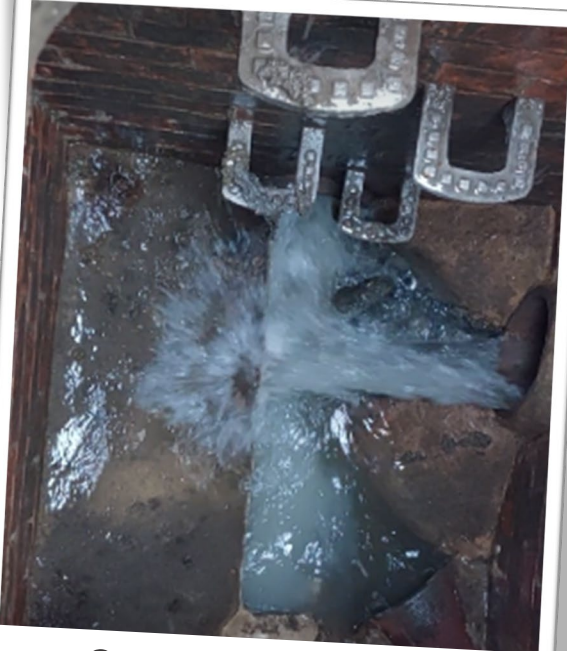
Gurnard, Isle of Wight Large illegal surface water connection
